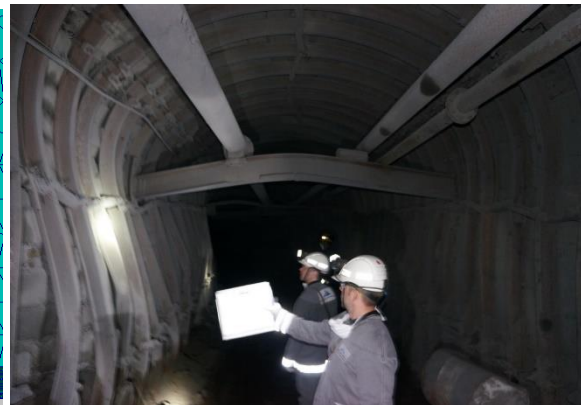
Reinforcement (tamponage) + Replacement of SVP 27 at SVP 33 Horizontal convergence 30 cm
